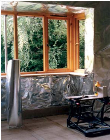
Eco-Brite being installed in a private home prior to fitting plasterboard
