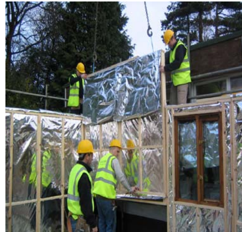
Eco-Brite installed in prefabricated wall panels
