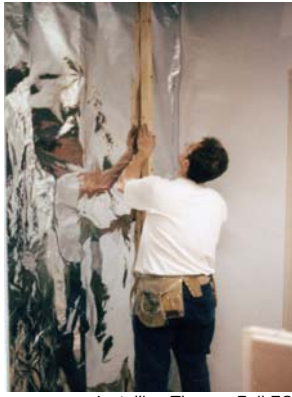
Installing Thermo-Foil ES
