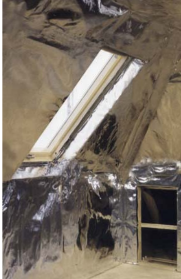
Thermo-Foil ES being installed in a private home prior to fitting plasterboard
