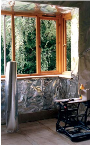
Eco-Brite being installed in a living area prior to fitting plasterboard
