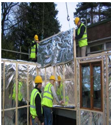
Eco-Brite installed in pre-fabricated wall panels
