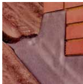
Chimney flashing – Grey finish
