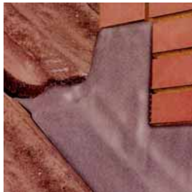
Chimney flashing – Grey finish
