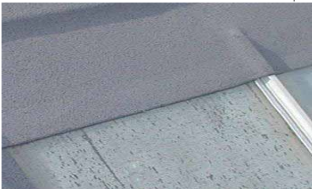
Flashing below window – Black finish
