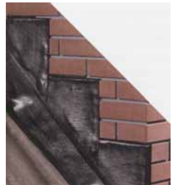
Chimney flashing –Black finish
