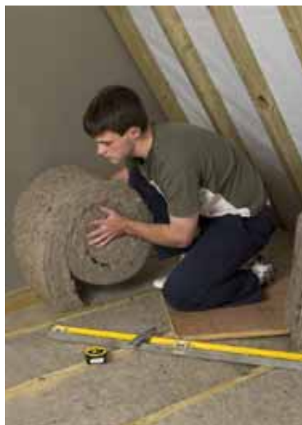
Installing ThermaFleece PB20 in a new home
