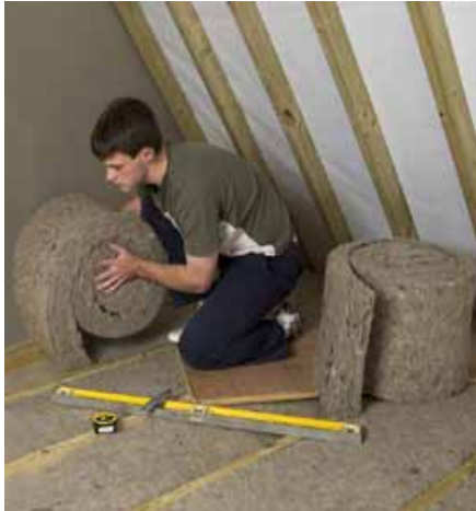
Installing ThermaFleece PB20 in a new home
