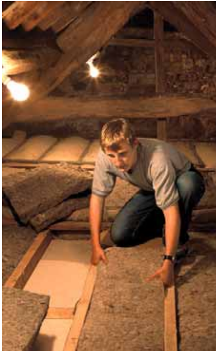
Installing ThermaFleece in a new home
