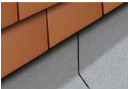
Ubiflex Grey below tile façade flashing
