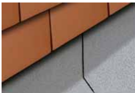
Ubiflex Grey below tile façade flashing
