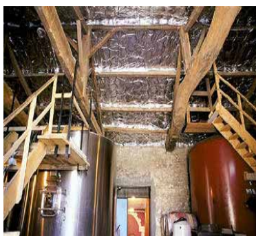
TRI-ISO SUPER 10 Under rafter application
