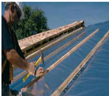
TRI-ISO SUPER 10 Installed prior to fitting roof tiles
