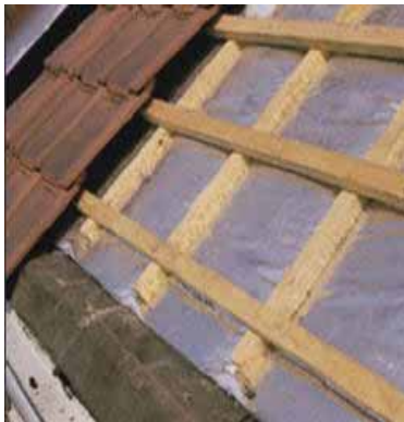
TRI-ISO SUPER 10 installed prior to fitting roof tiles
