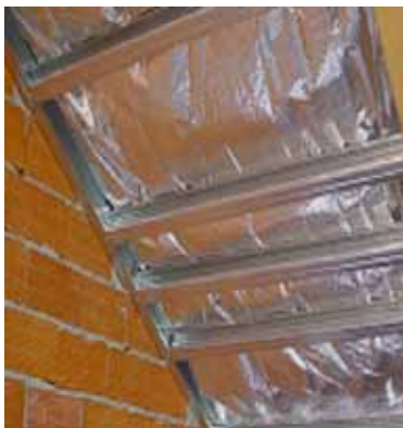
TRI-ISO SUPER 10 Positioned under rafters
