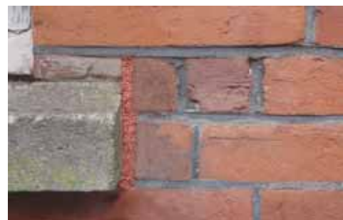
FLEXIM® GF adhesive mortar resists expansion and contraction, stays flexible, never cracks or loosens and never falls out.
