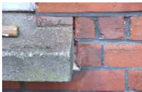
Most proprietary fillers in this sort gap will shrink, expand, crack, loosen then fall out!
