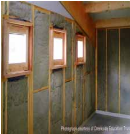
Installing ThermaFleece in a new home
