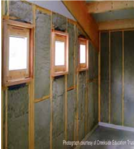
Installing ThermaFleece in a new home
