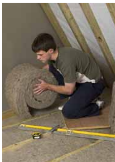
Installing ThermaFleece PB20 in a new home
