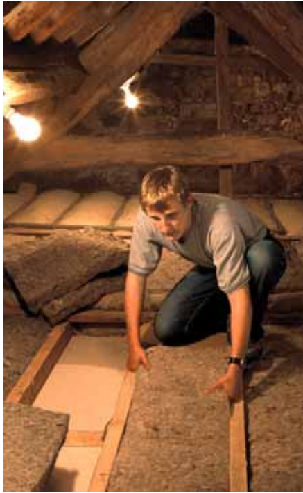
Installing ThermaFleece in a new home
