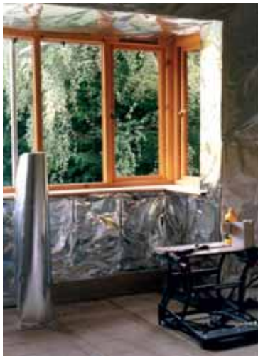
Apollo HPA adhesive tape being used to seal a Heat Reflecting Membrane installed in a private home prior to fitting plasterboard
