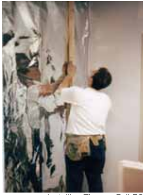
Installing Thermo-Foil ES
