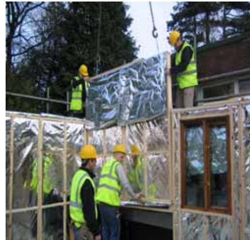
Eco-Brite installed in prefabricated wall panels
