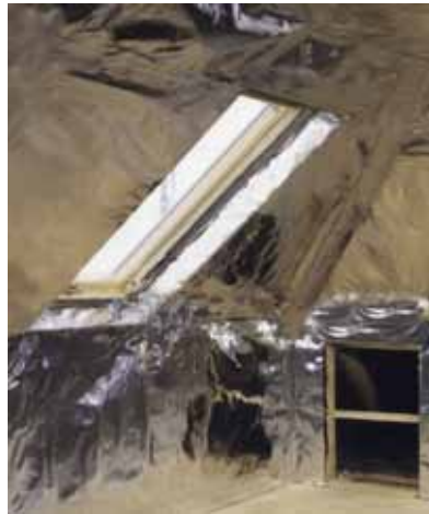
Thermo-Foil ES being installed in an attic room prior to fitting plasterboard
